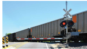
Illinois, Ohio panels OK funds for grade crossing safety projects
